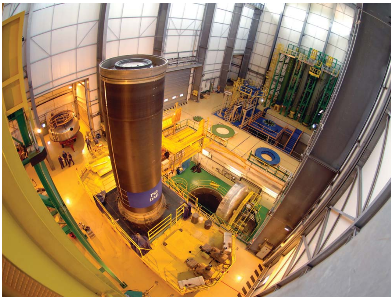
The Vega P80 motor in the Guiana Propellant Plant (UPG) in Kourou (Fr. Guiana) in September (Photo: ESA/CNES - P. Baudon)
