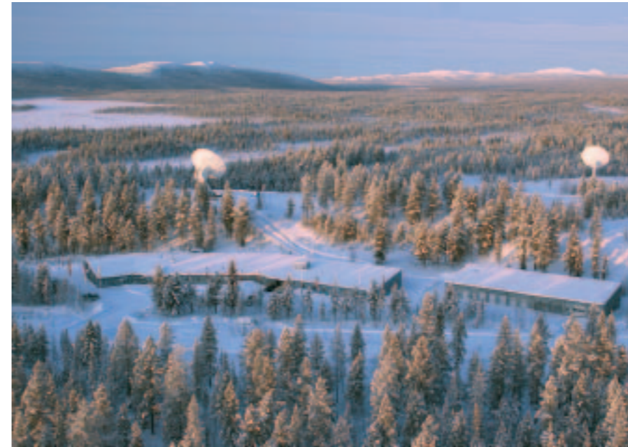
The ESA Kiruna ground station, originally set up for ERS-1, had a second antenna added for Envisat. As well as supporting other ESA missions, it is the only ground station for the CryoSat mission and hosts the data-processing, local-archiving and distribution functions
